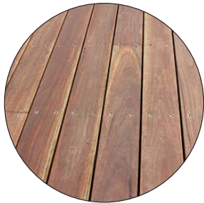
[P06] BOARDWALK 150mm wide hardwood decking screwed to timber frame
