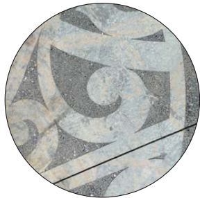
[SB1] CONCRETE TYPE 3. SANDBLAST CONCRETE PATTERN Stencil sandblast concrete to medium depth 2mm, to show patterns
