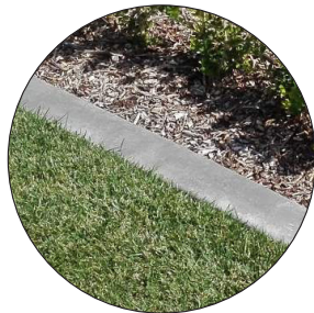
[E02] CONCRETE EDGE 150mm thick, centrally reinforced, on 150mm compacted AP40. Concrete strip to edge lawn to garden bed/hoggins and tiger turf
