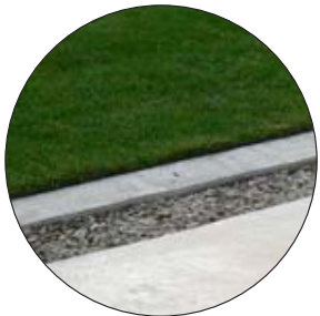
[E01] CONCRETE NIB KERB 200mm wide, smooth steel float finish with 5% black oxide pigment.
