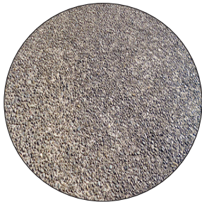
[P02] CONCRETE TYPE 2. EXPOSED AGGREGATE CONCRETE Local 10mm chip with Peter Fel coloured concrete (colour TBC) Pedestrian: 110mm thick, reinforced on 100mm compacted AP40
