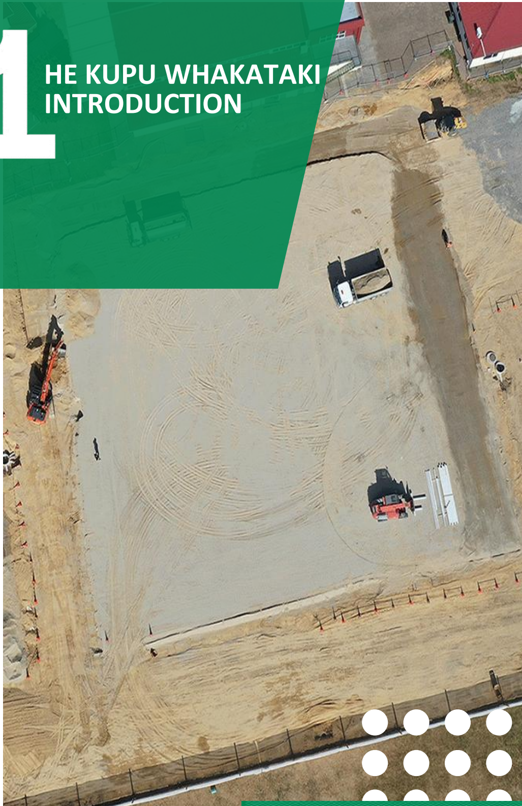
Photo of: Open Stadium Matamata development
