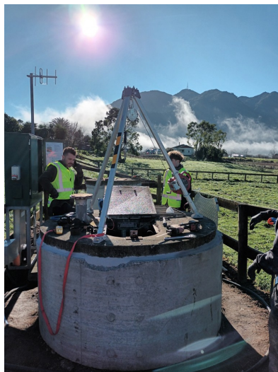
← Confined space entry at Turley Sewer Pump Station, demonstrating an engineering control, a tripod and winch system providing safe access/egress.
